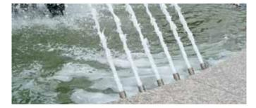
Smooth bores are great, they are the most versatile and effective jets to create clear-water streams and especially now with the integral flow straighteners they are unbelievably efficient. Sometimes though, smooth bores are just not enough.
